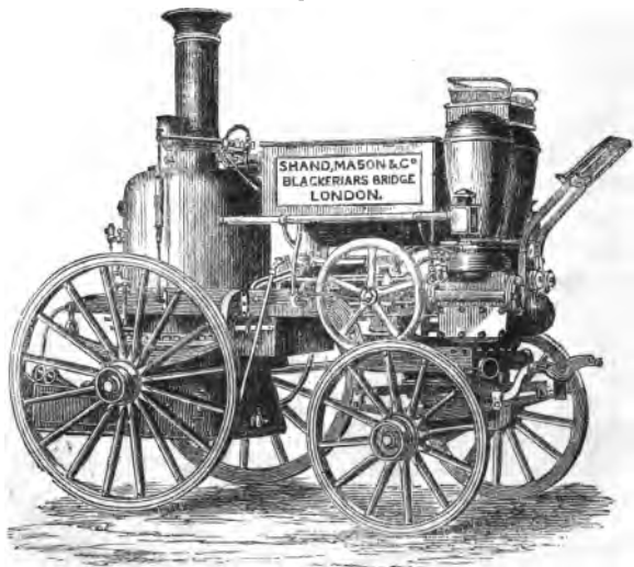
SHAND, MASON AND Co.'s HORIZONTAL STEAM FIRE-ENGINE.
